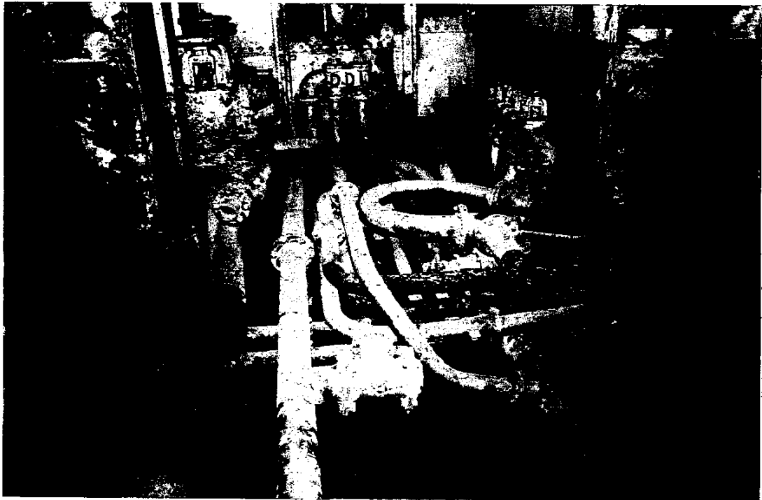
PART OF BILGE PIPING SYSTEM
