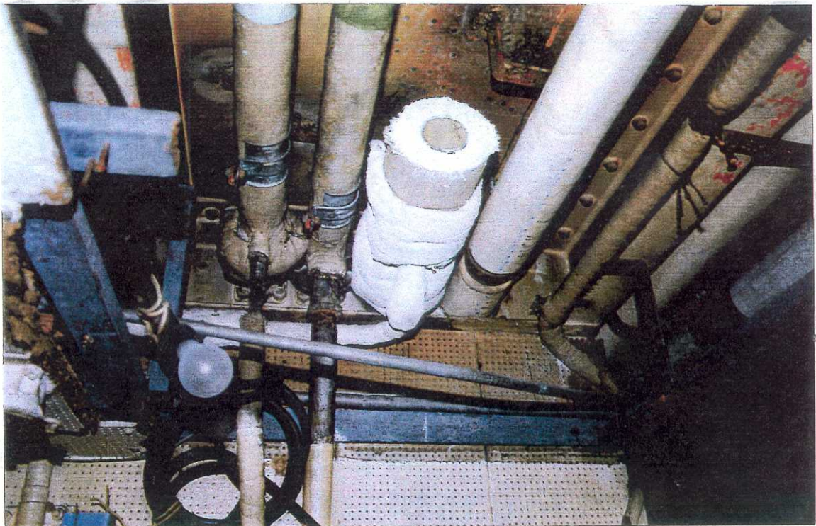
TYPICAL PIPE LAGGING "C" DECK WORKSHOP, PORT SIDE
