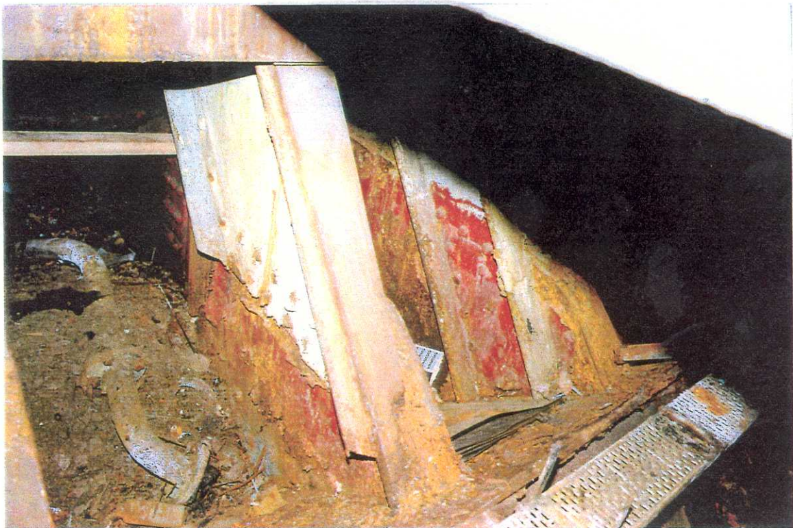
SHAFT BILGE AREA, STBD SIDE
