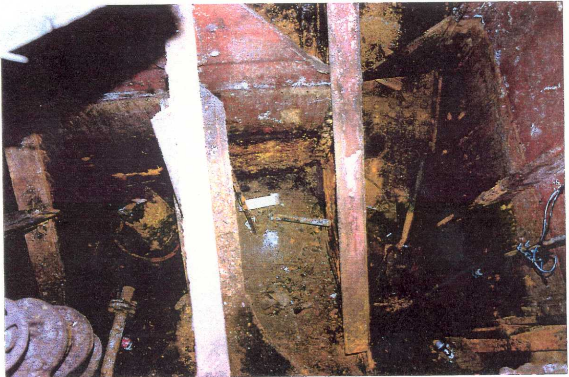
BILGE DETERIORATION CENTERLINE / AFT
