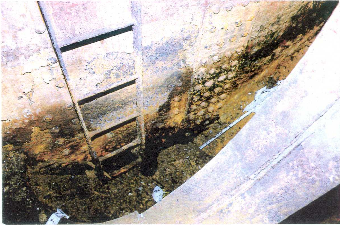
BILGE AREA, PORT SIDE, AFT
