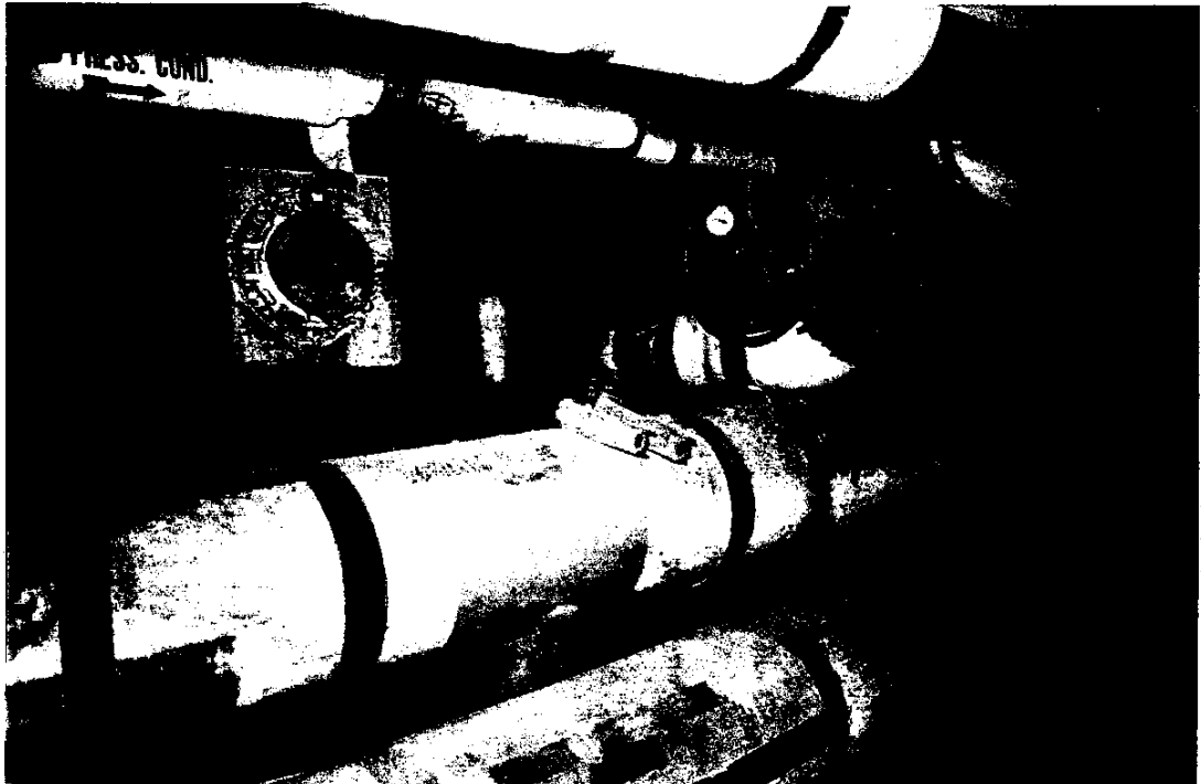
PENETRATION POINT FOR MAIN STEAM LINE ENTERING SHIP
